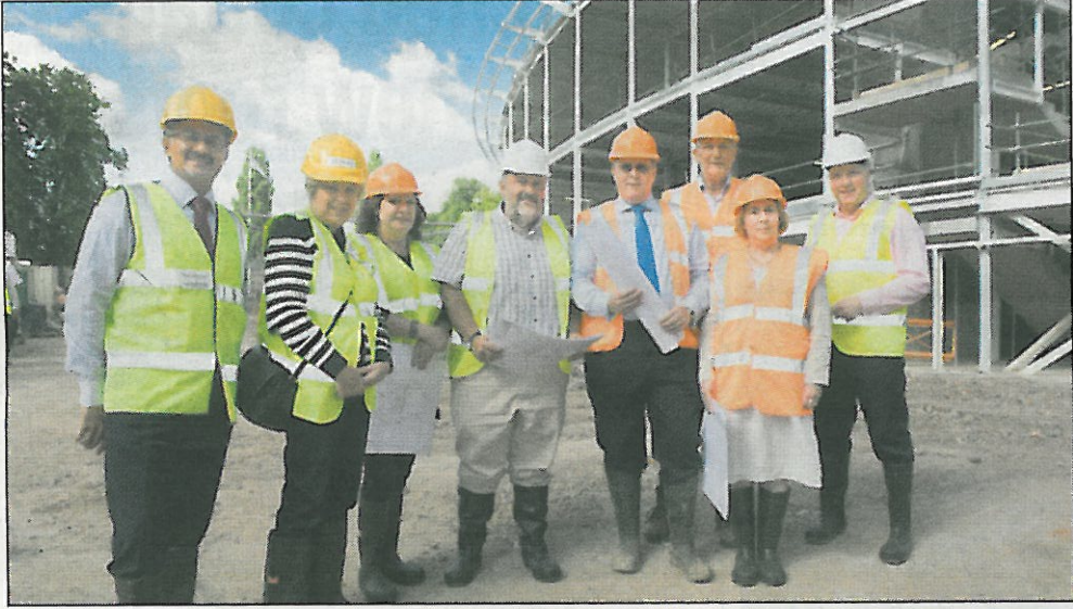
At the topping-out ceremony are (left to right): Sanjiv Kohli (Borough Council Deputy Chief Executive for Corporate Direction), Councillors Maureen Cook, Jan Kirby, Ozzy O'Shea and Russell Roberts, Peter Kirkham (MD of Places for People Leisure), Cllr Miriam Surtees and Bill Cullen (Borough Council Deputy Chief Executive for Community Direction).
